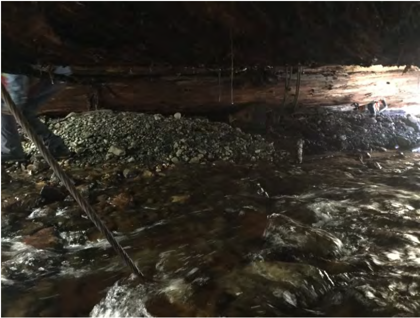
Left Bank Abutment when facing downstream
